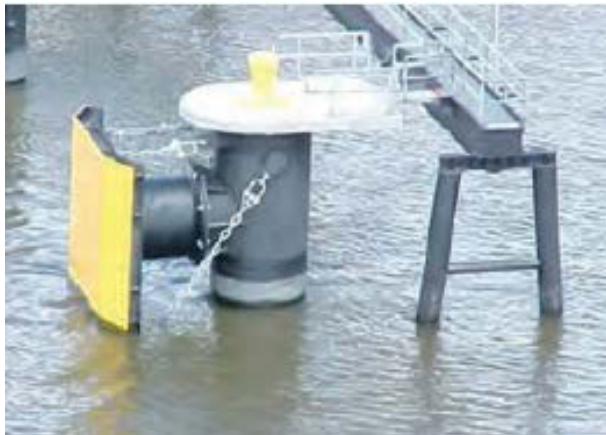
Figure 12-4: Mono-pile breasting dolphin (typical)
