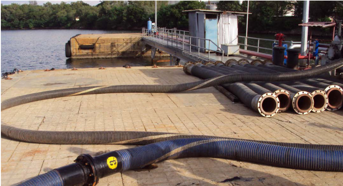
Figure 12-1 Oil Jetty - Central Platform
