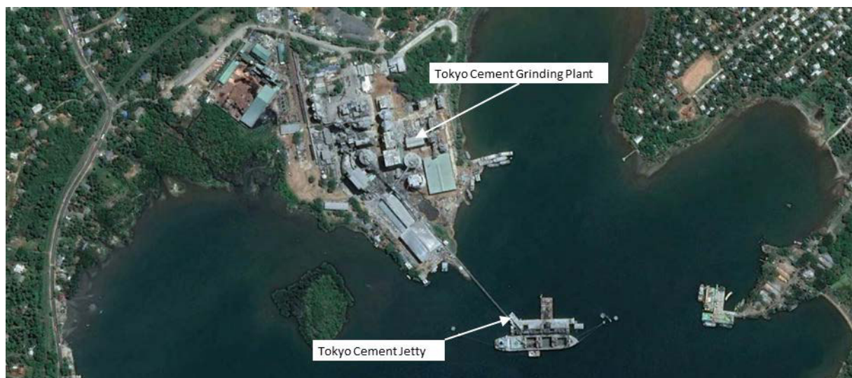
Figure 2-4: Tokyo Cement Facility
