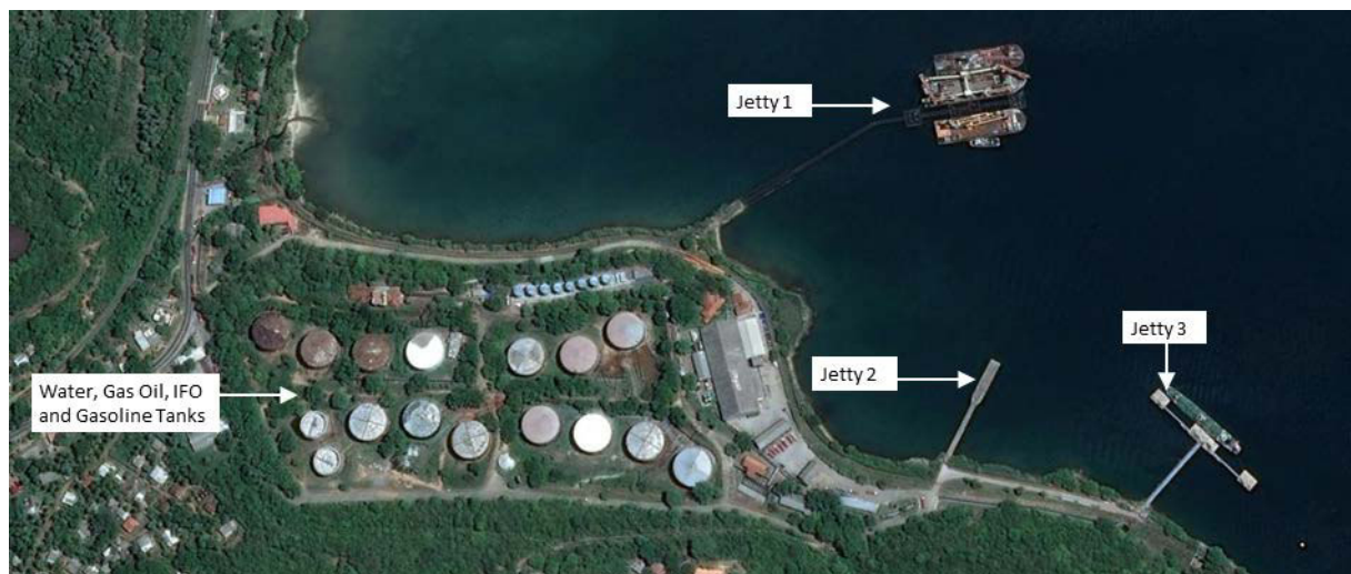
Figure 2-6: Lanka IOC Facility and SLPA's jetties
