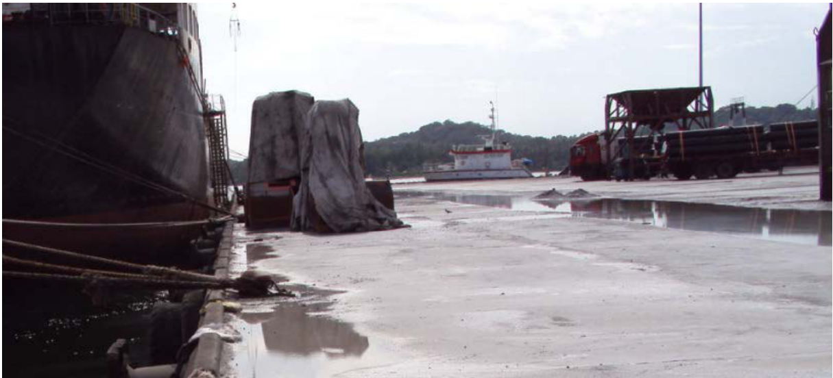
Figure 11-4: Quay Alignment and Water Accumulation
