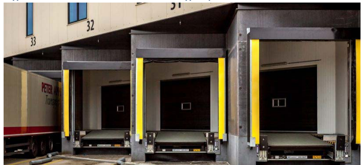
Figure 9-1 Warehouse Truck Loading Bays
